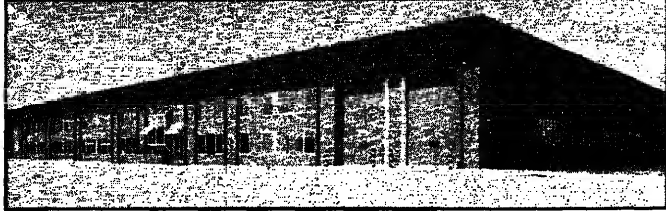
Aquascutum of London, the clothes makers, have acquired this 39,000 sq ft property on the Maylands Estate at Hemel Hempstead. The company has taken a full repairing and insuring lease from Brixton Estate for 25 years at close to the asking rental of £3.50 a sq ft. The move enables this long established manufacturer to meet its needs in the 1980s
